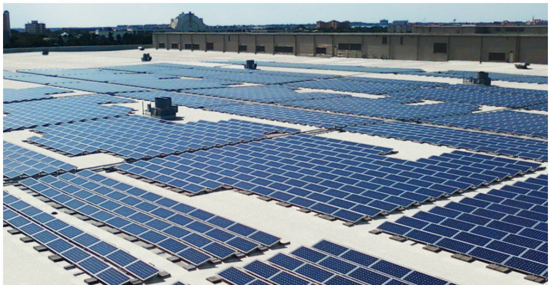
FiberTite Roof Orlando Convention Center
